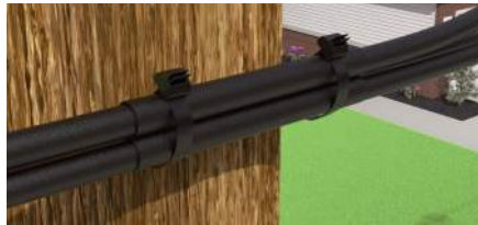
Cable Abrasion Protectors Installed on Cables
