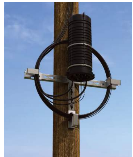
COYOTE® 9.5" x 28" Terminal Dome Mounted on 33" Fixed Crossarm Vertical SLACKLOOP System
