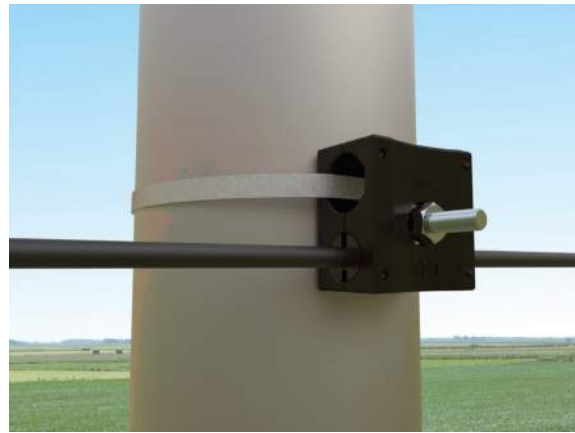
Lite Support Banded to Pole
