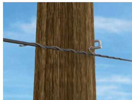
Standard Tangent Support with Flat Drop Cable
