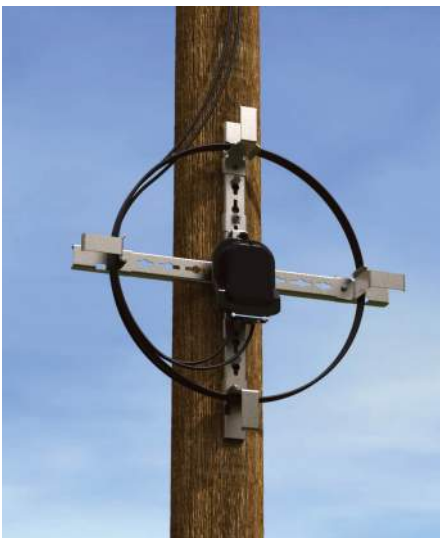
COYOTE® DTC8 Mounted on 33" Fixed Crossarm Vertical SLACKLOOP System
