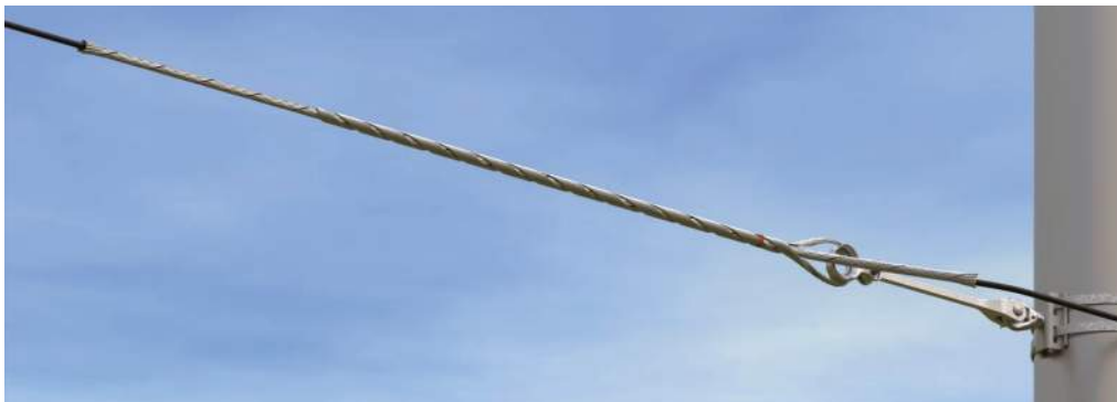
FIBERLIGN Medium Tension Dielectric Dead-End Installed on Steel Pole with Thimble Clevis, Extension Link, and Banding Bracket
