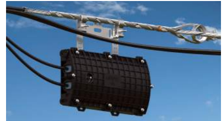
COYOTE® In-RUNT Mounted to Dead-End
