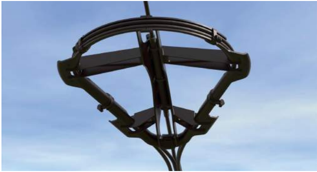
Cable Installed in Center-Lock Storage Bracket with Filler Tubes
