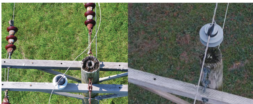
The drone inspection conducted by PLP discovered severe rot on the top of several poles.
